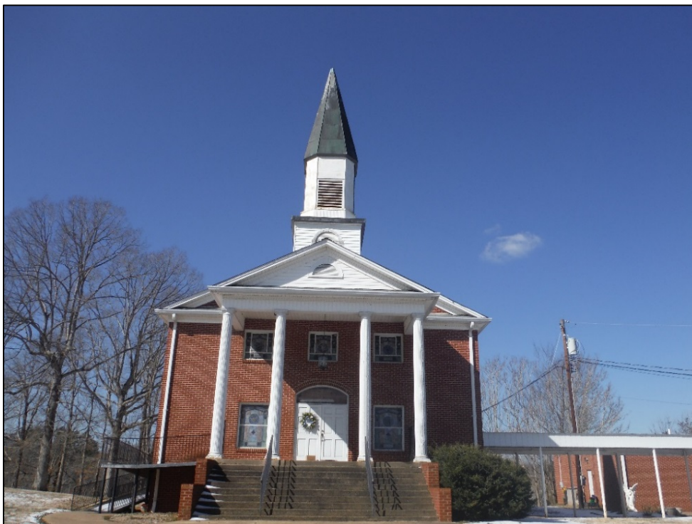
Figure 3. View of Buffalo Baptist Church, facing west.
