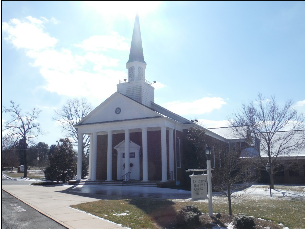
Figure 18. View of Fallston Baptist Church, facing south.
