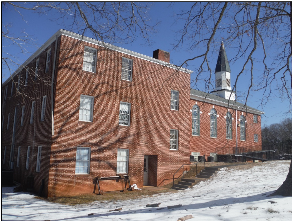
Figure 6. Rear oblique of the Buffalo Baptist Church, showing annex, facing northeast.
