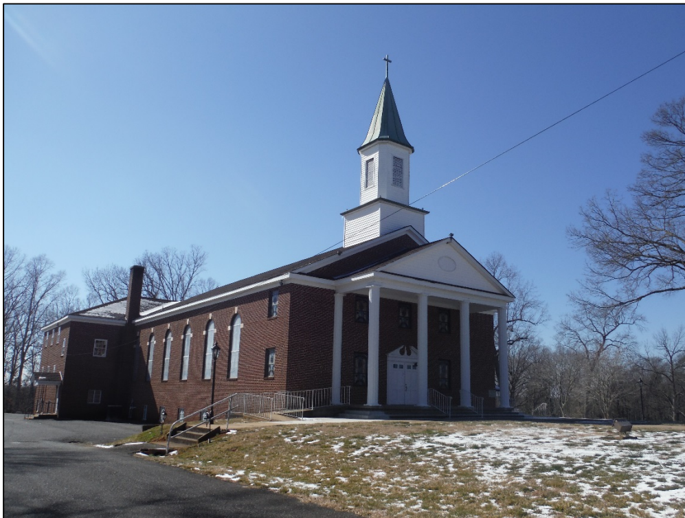
Figure 23. View of Sandy Run Baptist Church, facing southwest.
