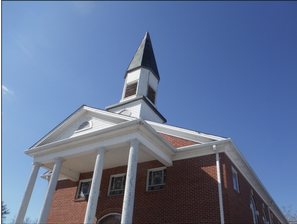
Figure 7. View of portico and steeple of the Buffalo Baptist Church, facing southwest.
