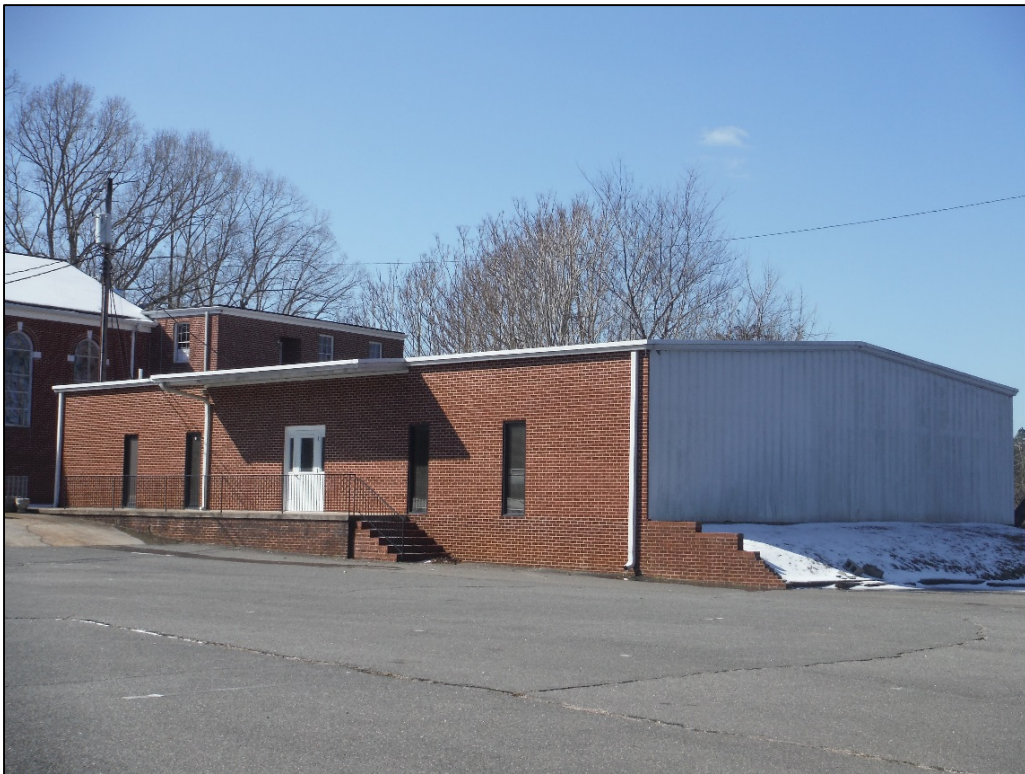
Figure 15. Oblique view of Fellowship Hall I building associated with Buffalo Baptist Church, facing southwest.
